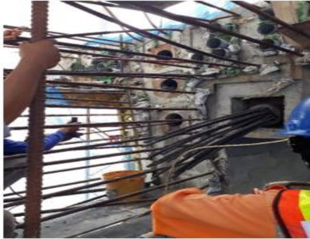
Gambar 4.47. Pipa tendon tersumbat beton coran
