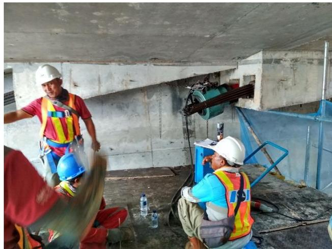
Gambar 4.46. *Stressing tendon box girder*
