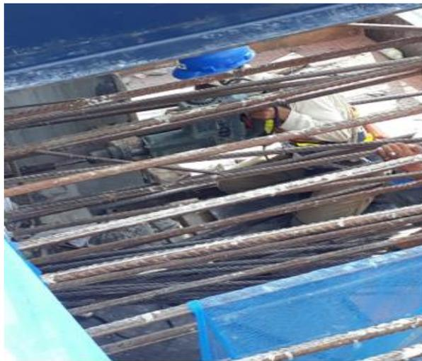
Gambar 4.49. *Coring* pipa tendon
