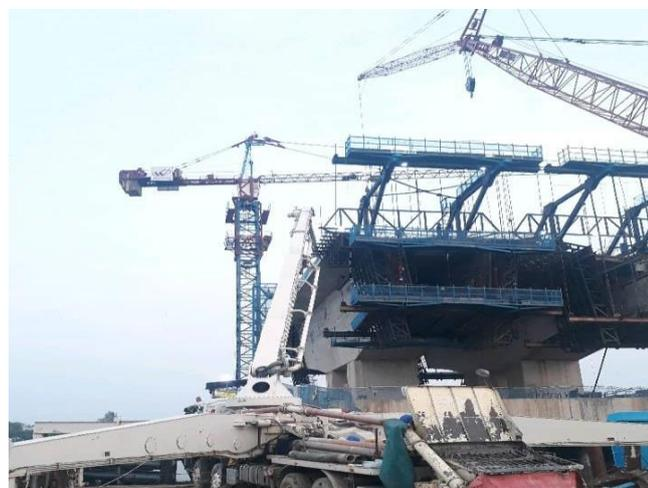
Gambar 4.21. *Concrete pump*
