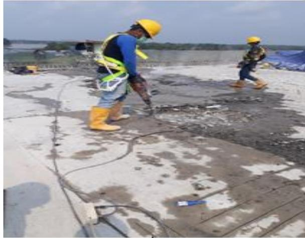
Gambar 4.48. *Chipping* beton
