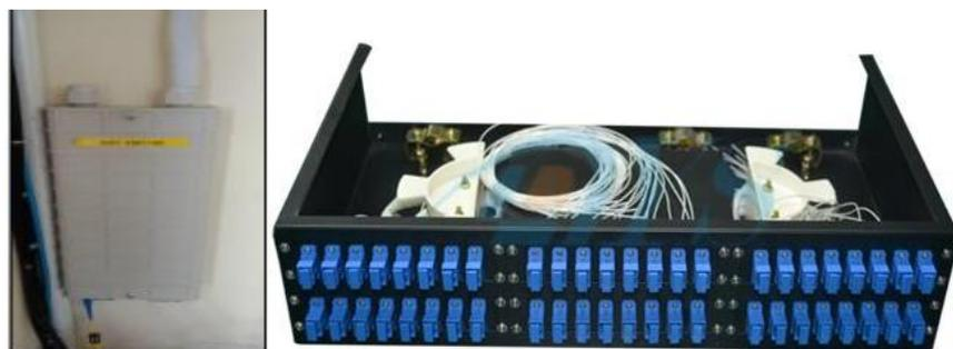
Gambar 3.3 *Optical Distribution Frame (ODF)*
