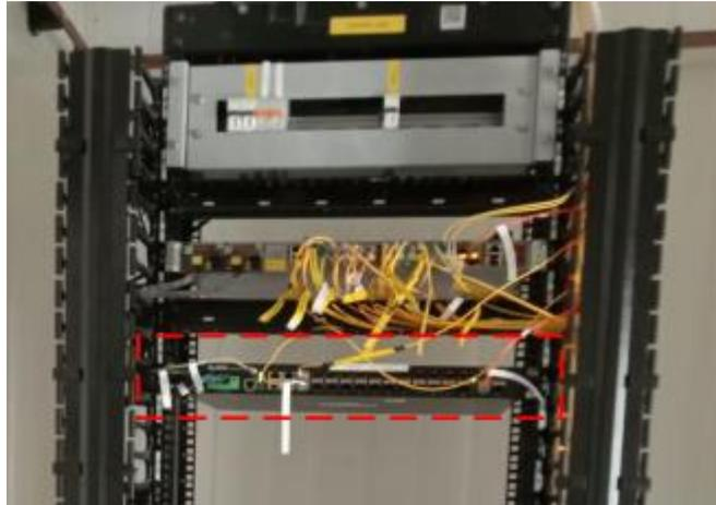
Gambar 3.6 Switch MGS3520
