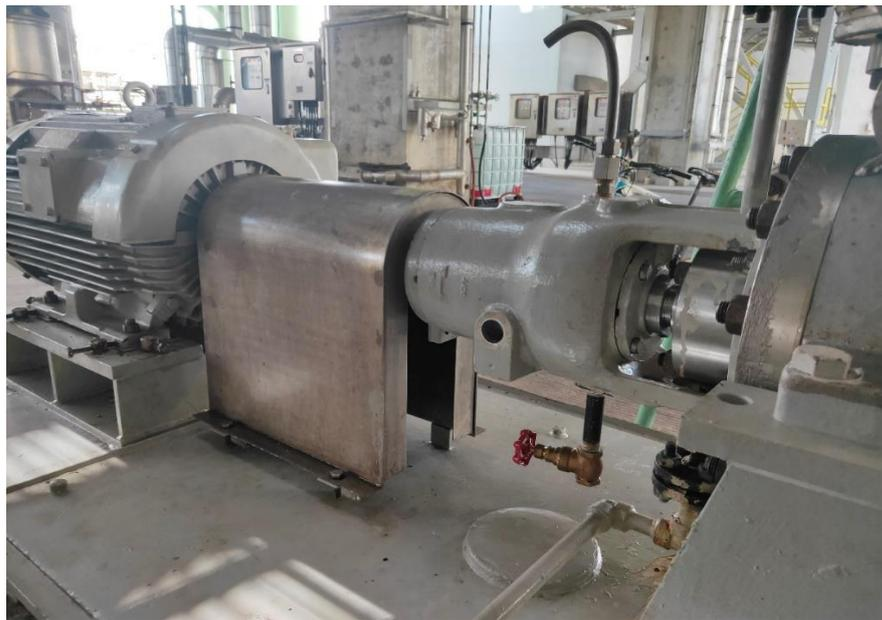
Gambar 1.1 Pompa Centrifugal Urea
