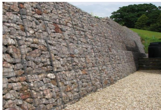
Gambar 3.4. Gabion Retaining Wall
