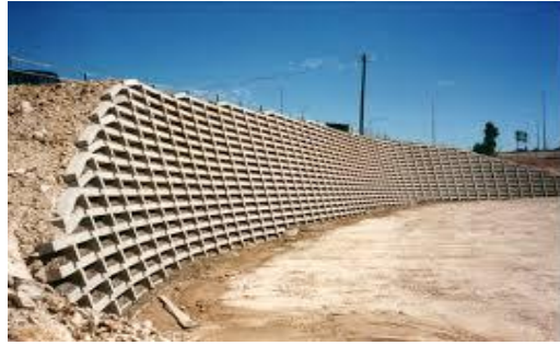
Gambar 3.3. Crib Retaining Wall
