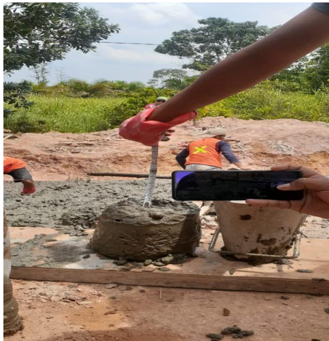
Gambar 4.1. Slump Test Beton
