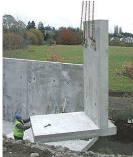
Gambar 3.5. Cantilever Retaining Wall
