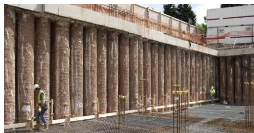
Gambar 3.8. Piled Retaining Wall
