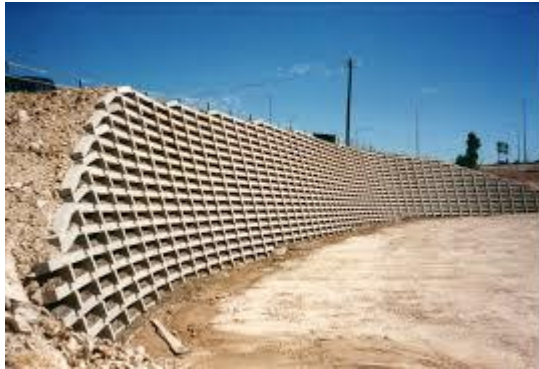
Gambar 3.3. Crib Retaining Wall
