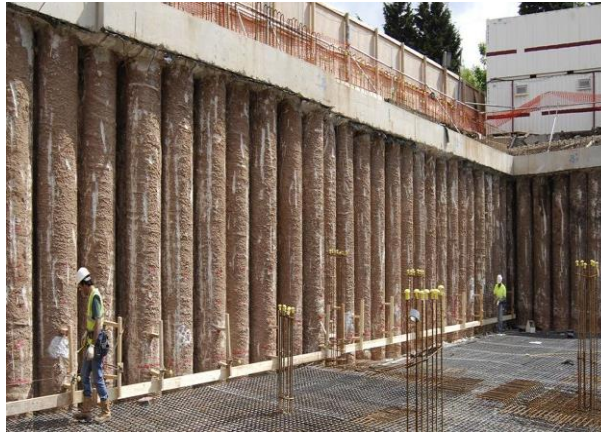
Gambar 3.8. Piled Retaining Wall
