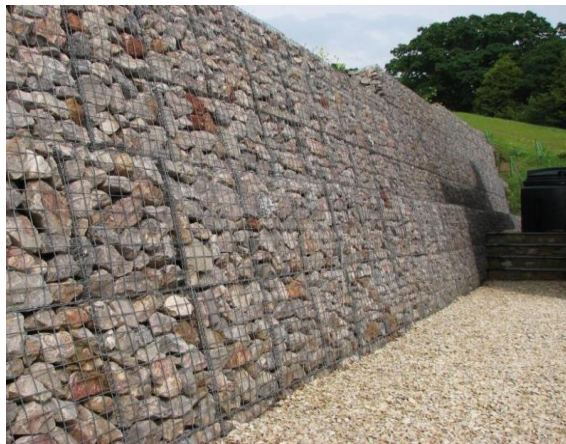
Gambar 3.4. Gabion Retaining Wall
