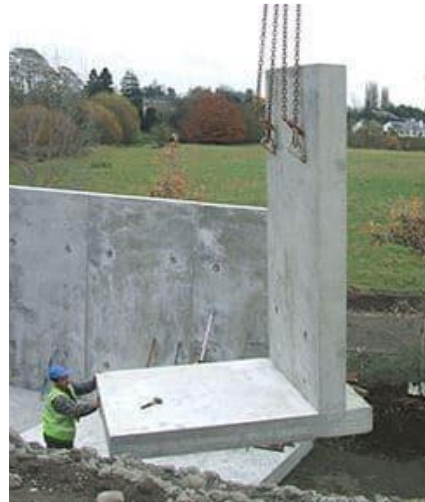
Gambar 3.5. Cantilever Retaining Wall
