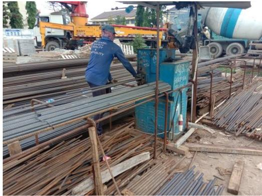
Gambar 4.6 Alat Pemotong Besi ( *Cutting Bar* )
