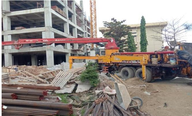
Gambar 4.4 *Concrete Pump*
