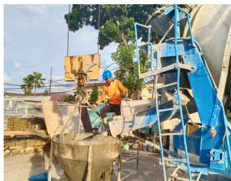
**Gambar 3.14** *Concrete bucket*
