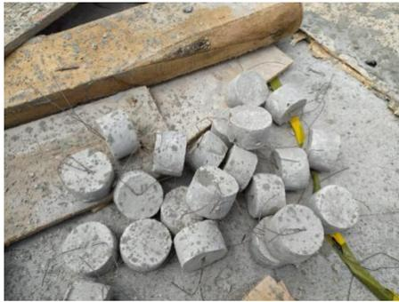
**Gambar 3.29** Beton Decking
