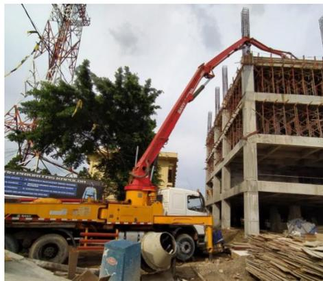
**Gambar 3.13** *Concrete Pump*
