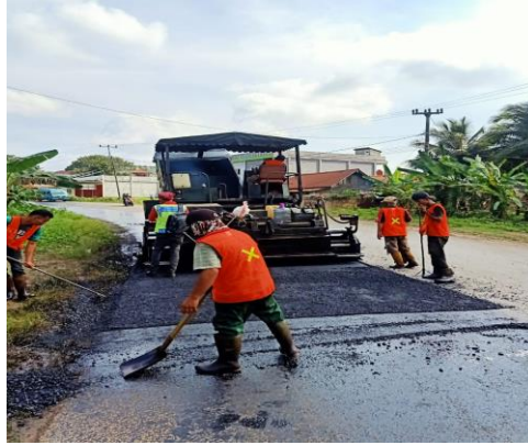
Gambar 4.6 Proses Pelekatan Tack Coat
