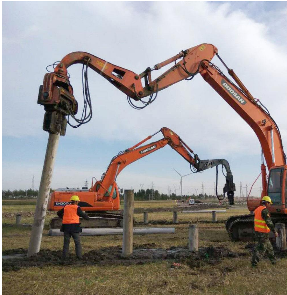
Gambar Vibratory Pile Drive
