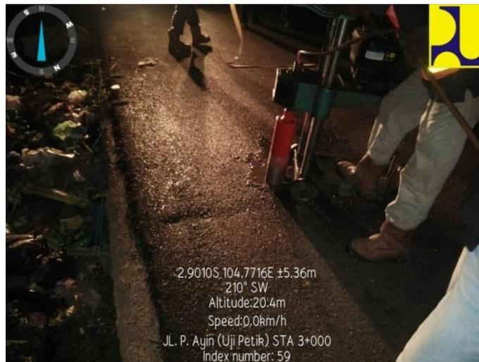
*Gambar 3.12 Core Drill*
