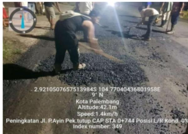
Gambar 4.3 Peghamparan agregat Titik Patching
