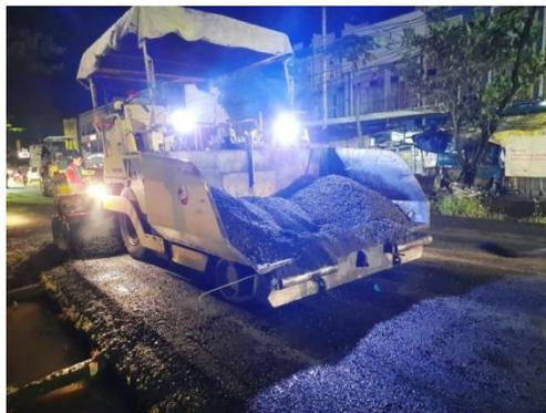
*Gambar 3.11 Asphalt Finisher*
