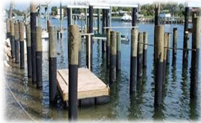
Gambar 3.4. Tiang Pancang Water Proofed Steel Pipe And Wood Pile
