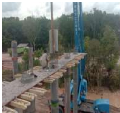
Gambar 4.2 (A) Cut of Pile
