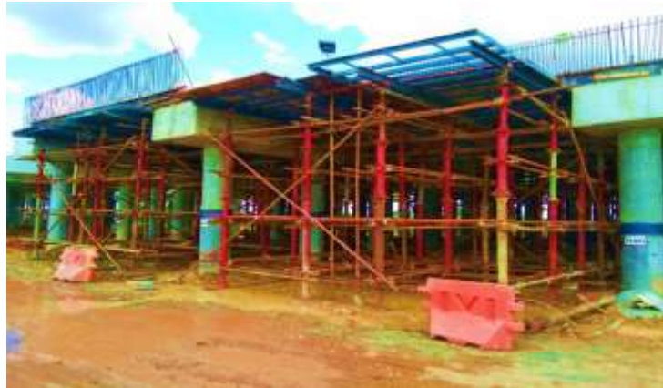
Gambar 3.9 Scarfolding/Tiang Perancah
