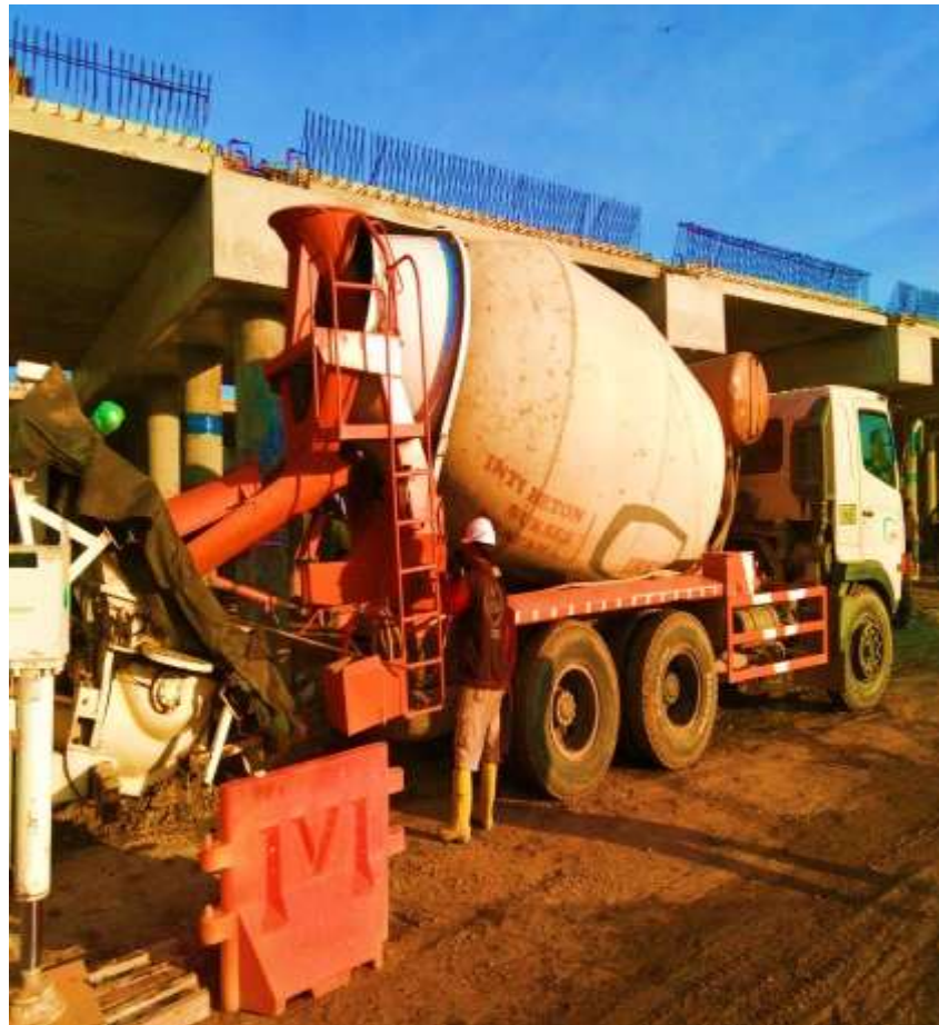
Gambar : 3.2 Truck Mixer Beton
