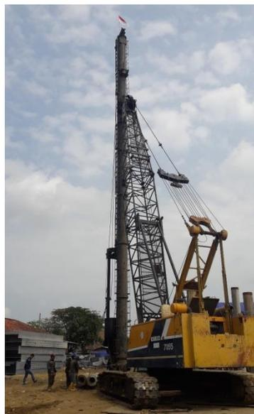
Gambar 4.2 *Diesel Hammer*
