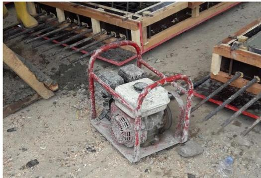
Gambar 4.7 *Concrete Vibrator*
