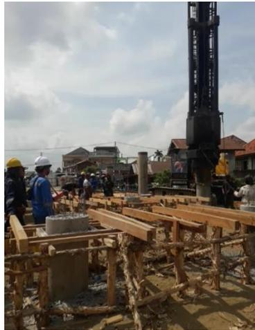
Gambar 5.4 Pengujian *Pile Driving Analyzer* (PDA Test)
