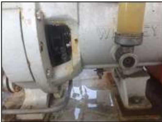
Gambar 1.1 Kebocoran Aluminium Sulfate
